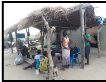
Photo 3a: Wooden shed with zana mat as roof, Bukasu fishing camp (Ghana)
