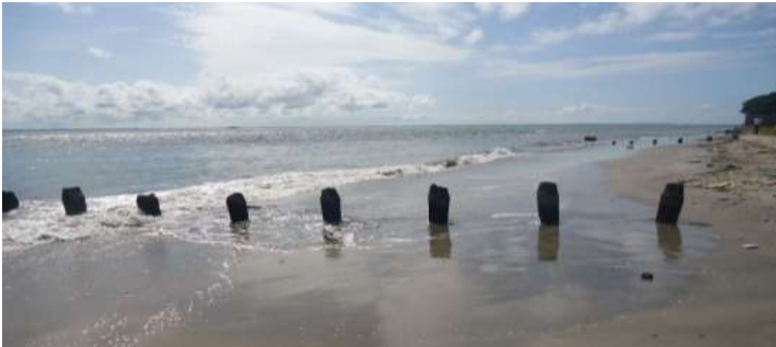
Figure 4. 5 Groyne system destroyed by coastal erosion and wave action
