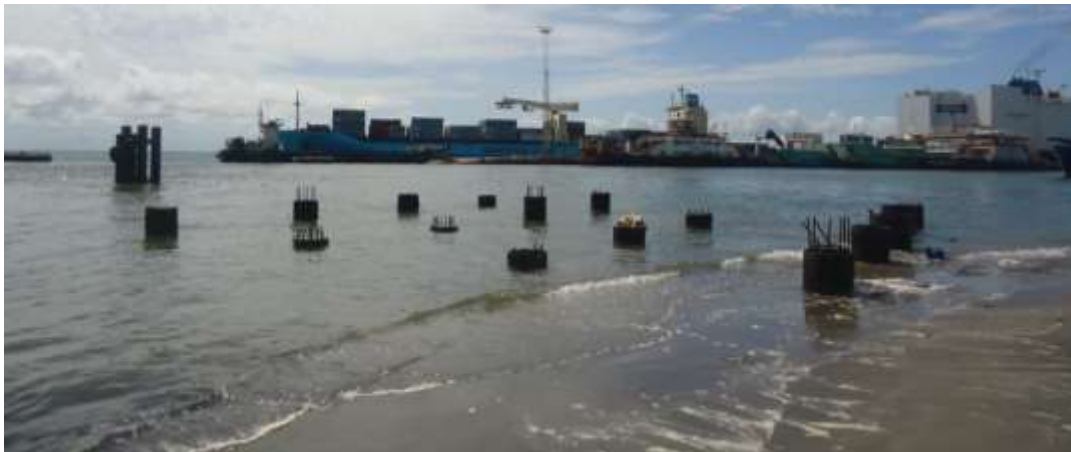
Figure 4. 6 Old Wharf destroyed by coastal erosion and wave action
