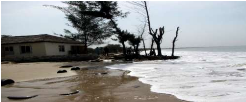
Figure 4.3 Some buildings at risk to coastal erosion
