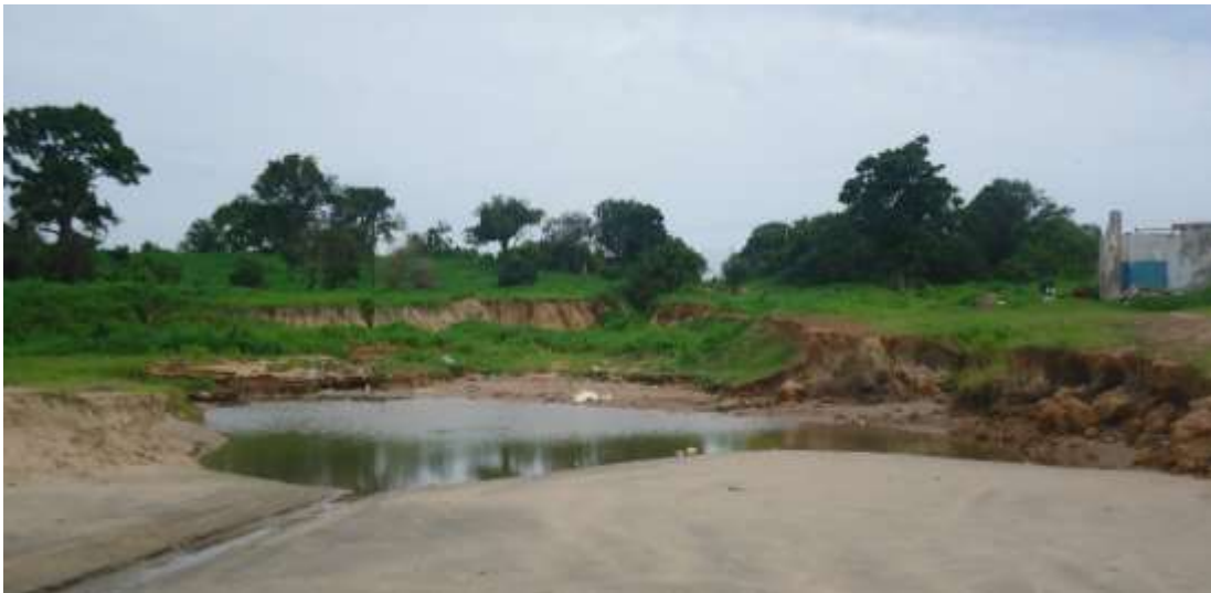
Figure 4. 15 Coastal Erosion along the Cell
