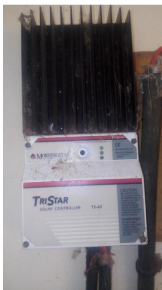
Figure 3-8: Photography of the charge controller connected
