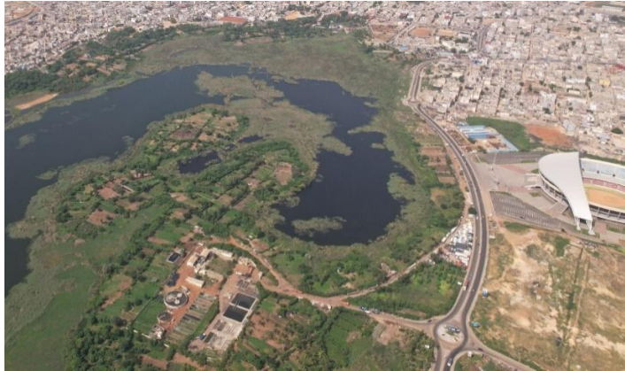
Plate XV: Buildings encroachment in the NURGND
