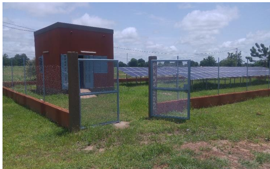
Figure 1: PV off grid in Digré
