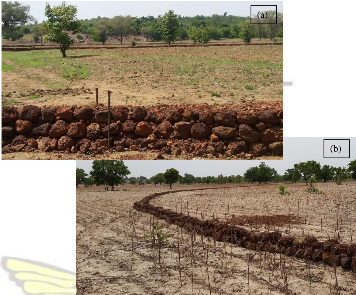
Figure 2-1: Stone bund constructed with lateritic duricrust on cropland in Manzour (a) and Dibogh (b) in the Ioba province of Burkina Faso. Images captured on 29 th May, 2017 during field visit.
