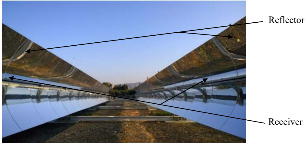
Figure. 5. 1. Collector of the first industrial PTC system in Cyprus [205], [209]
