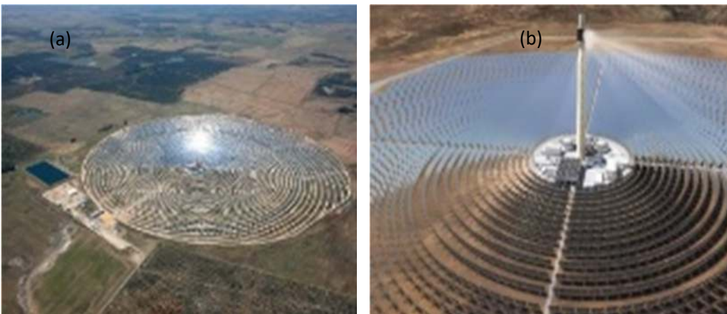
Figure. 1. 7. Gemasolar [33] (a) and Noor Ouarzazate III [39] (b) solar tower power plants
