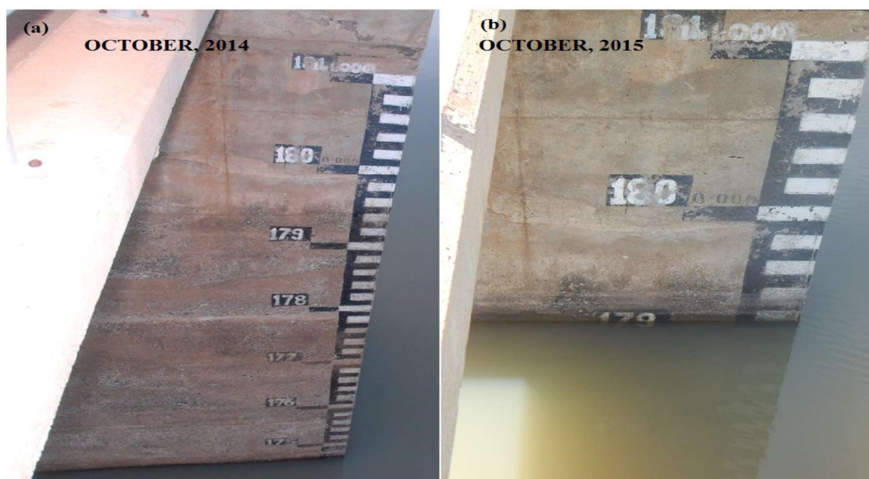
Plate 4.1 (a) Tono dam level using staff gauge, measurements in October, 2014 and (b) in October, 2015
