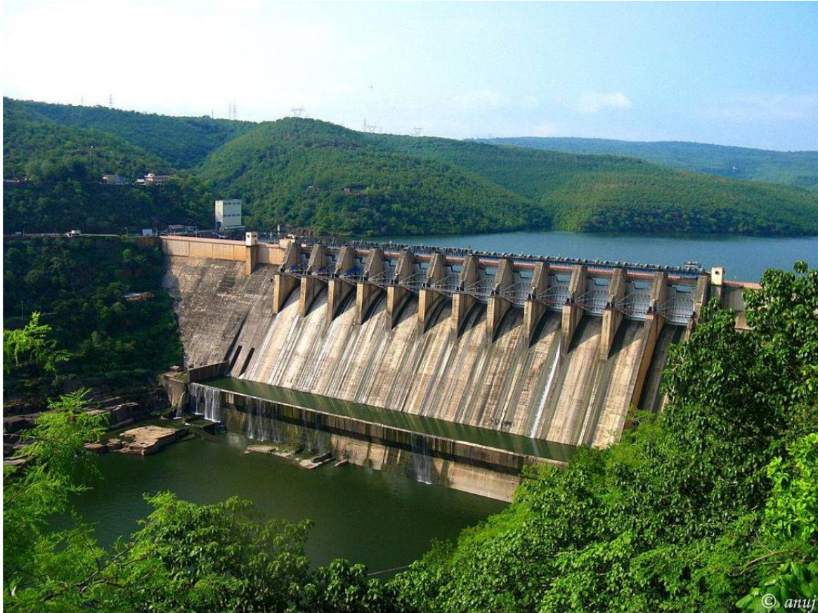
Figure 2 : GD-3 dam( https://infrastructurebrief.com/ethiopia-completes-construction-of-genale-dawa-iii-dam
