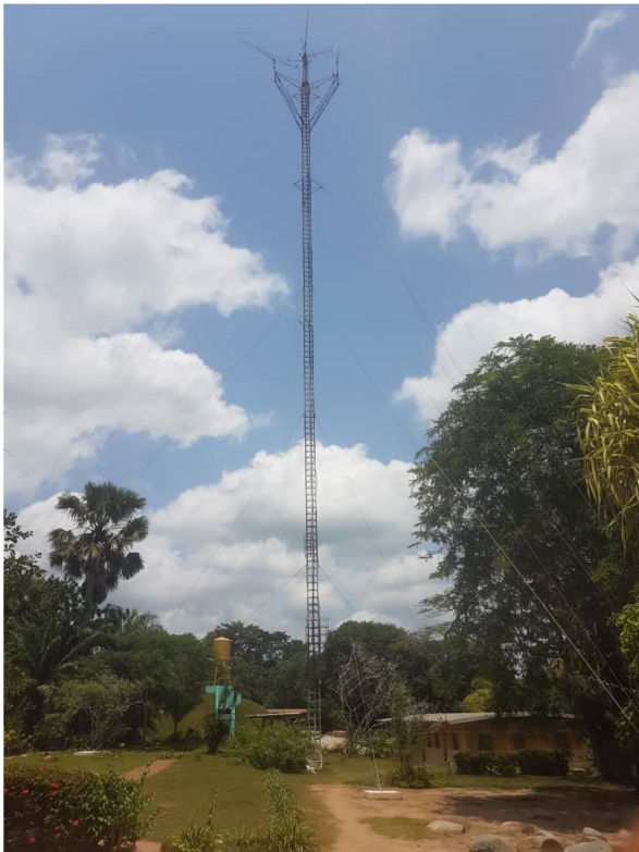
Fig. 4. View of the 50 m high tower. Meteorological sensors are installed at the top of the tower, together with the air intake.
